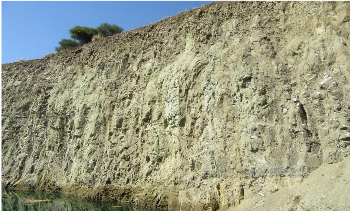
Figure 9.1 – Weathered pyroxenite highwall over the LG6 and 6A seams in the eastern mining area.
